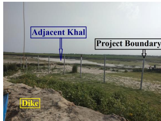
Dyke, Project Boundary and Adjacent Khal
