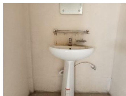
Wash Basin at The Dining Space
